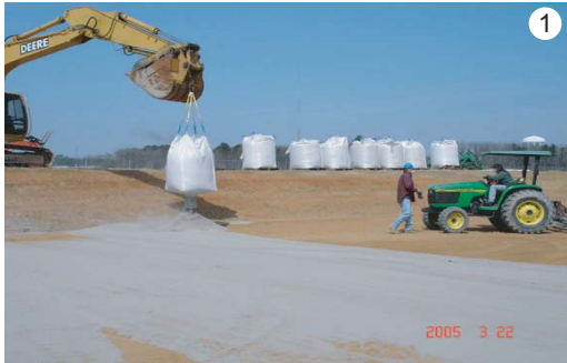
4. Mixing, placement of peat-amended biofiltration barrier
