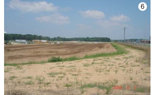
6. Nearly complete cell after placement of treated soils
