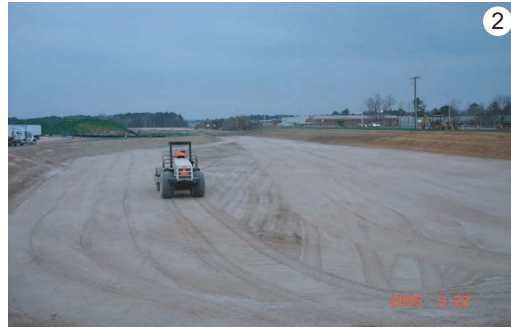
5. Placement of clean-soil berms to anchor GCL
