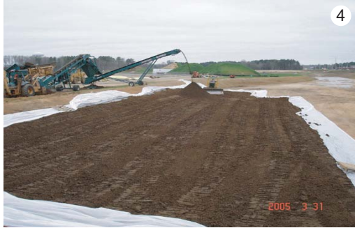
4. Mixing, placement of peat-amended biofiltration barrier
