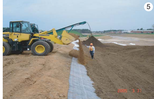
5. Placement of clean-soil berms to anchor GCL
