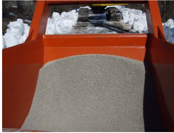
Figure 3: Organoclay Pellets ready for installation
