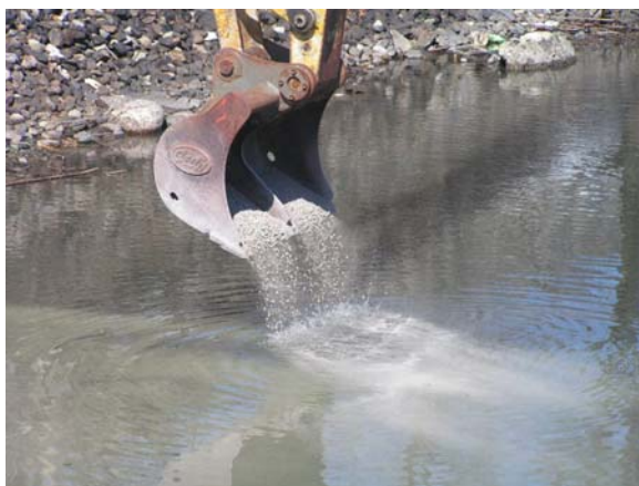
Figure 2: AquaBlok® + ORGANOCLAY™ Pellets being placed into water
